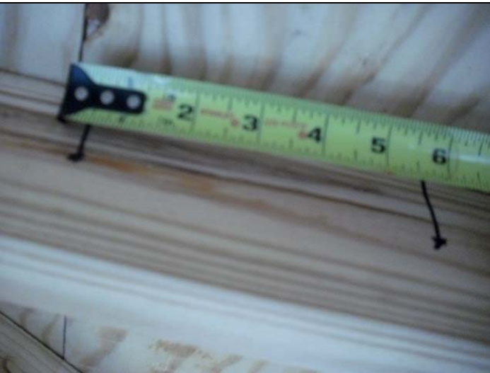
Roof deck attachment
