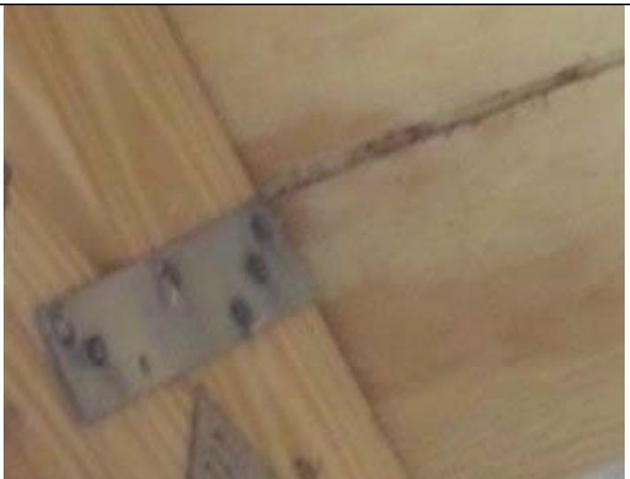
Roof to wall attachment
