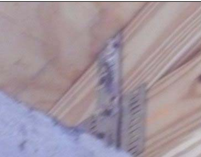
Roof to wall attachment
