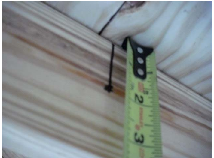
Roof deck attachment
